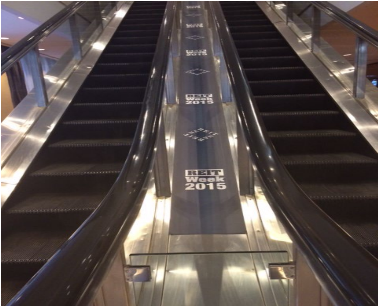
(1) West Escalator Runner – 3 rd floor to 2 nd floor (4) West Escalator Runner: Lobby to 2 nd Floor (5) Rhineland Gallery (Registration Area) to 3 rd Floor (Americas Hall) Escalator Runner
